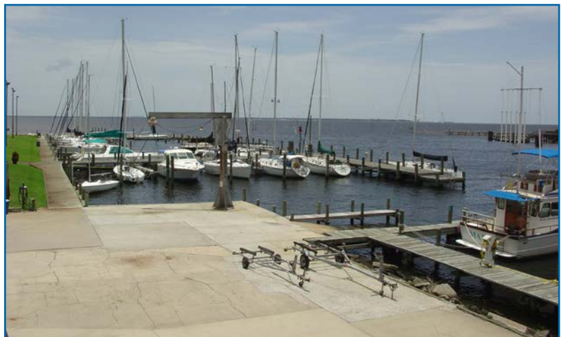
Repaired boat lift!
